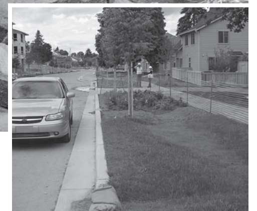
Photo by DAVIDE FERRO This planting bed along a major street in Seattle absorbs storm water, which relieves the combined sewer outfall of overflows caused by heavy rain.
